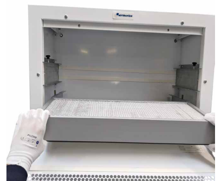
6- Remove the absolute filter pulling gently.
