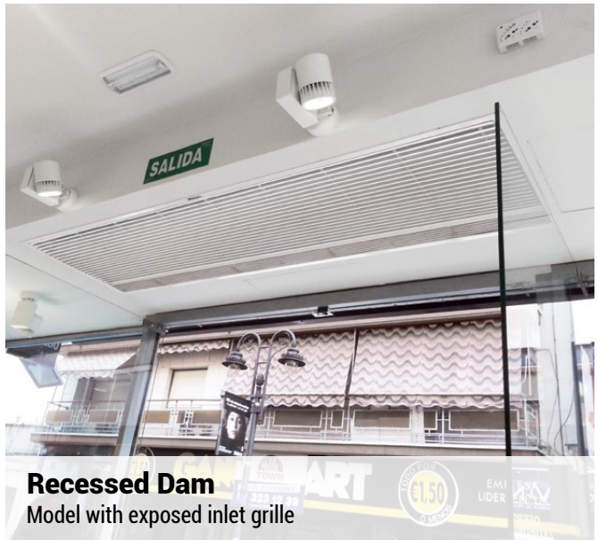
Windbox M,G Invisible installation with false ceiling kit
